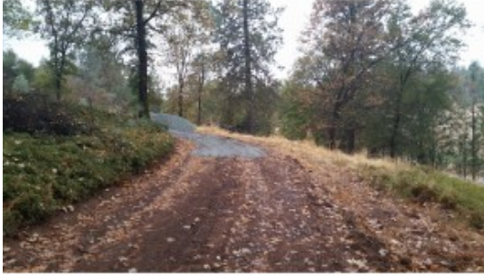
Gravel driveway going in CCAR 2017
